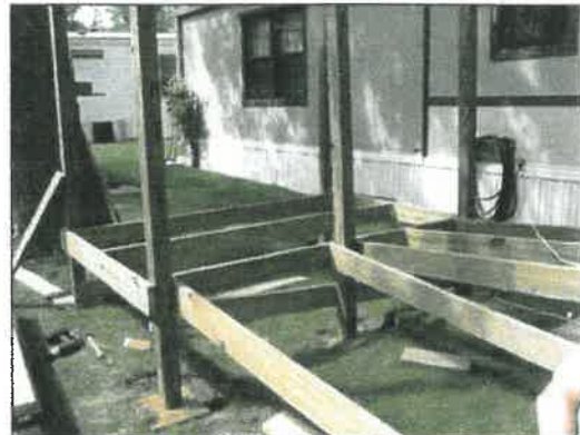
Figure 9. Ramp frame with 180° landing. Notice cross bracing
