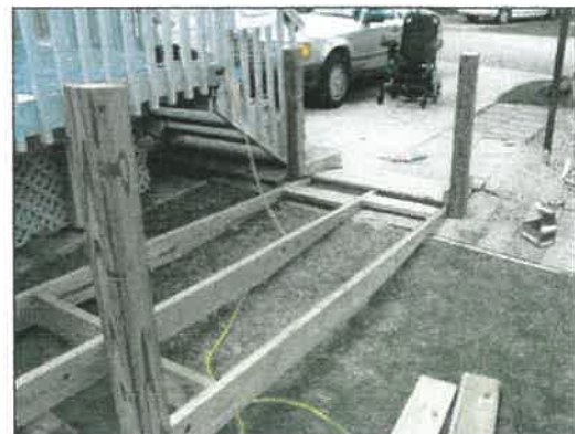
Figure 11. Stringers into Ramp end post assembly. Notice cross braces.
